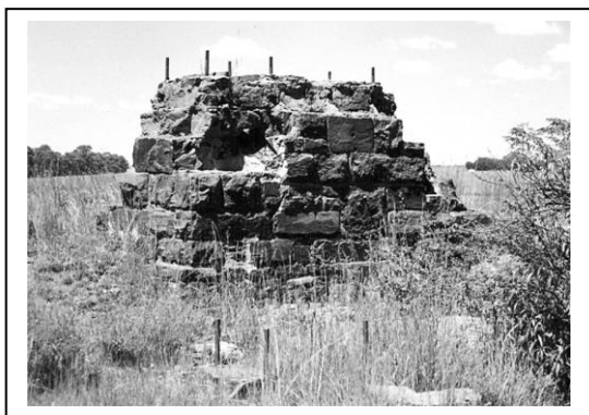
Fig 19 Blake jaw crusher foundation in 2008. 18
