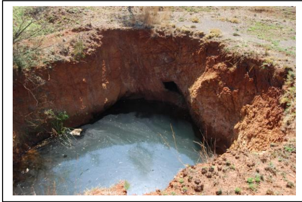
Fig. 9 Collapsed upper stope near winze E2.
