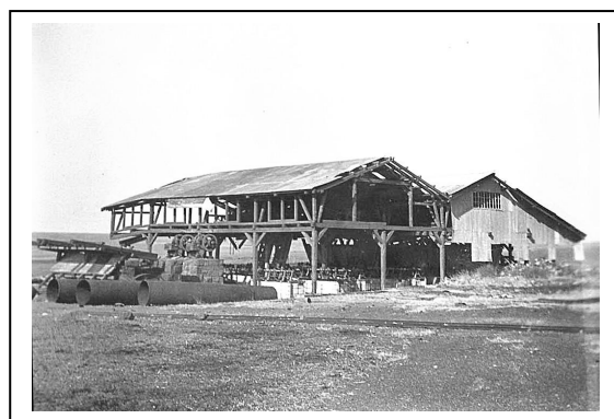
Fig 20 Blake jaw crushers & foundations in 1902 (they are just above the large pipes) with the 1890s concentration plant building behind. 19
