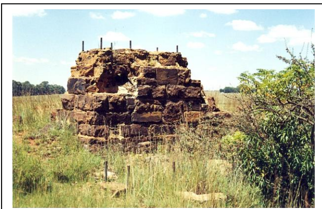
Fig. 13 Dry stone retaining wall in boiler house pit. Reuse of 1890s dressed stone.
